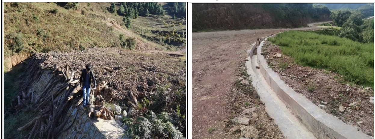
1#弃渣场浆砌石挡墙
